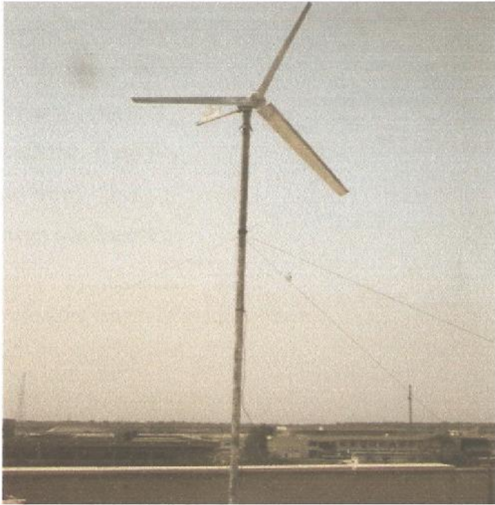
Fig.(3.1) wind turbine at AL-Khwarizmi collage of engineering
